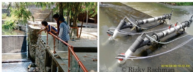
図 9 ガジャマダ大学の教官たちと彼らが作製したパイプ魚道 Fig.9 Instructors and a student of Gajah Mada University explained about the fishway at Candi Gebang Weir in Jogjakarta, Indonesia (left side), and siphon system pipe-type fishways that are installed another river near university for graduation research of that student (right side).
