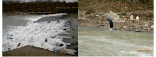
Fig.3 Slope with rubble for ascending fish (left) and inhabitant throwing a casting net (right) at a river in Giran Province.
