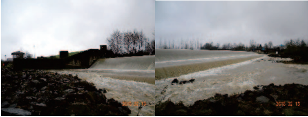
Fig.1 Pasikhan Dam at the Pasikhan River in Giran Province. The lift of this weir is 3.0m and its width is around 100m.
