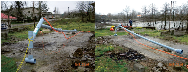
Fig.11 Fishway No.1 assembled at Pasikhan Dam in Gilan Province. This fishway is made of two parts with flange and able to be carried to setting site with truck.
